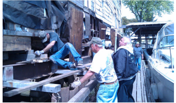
CONTINUING REPAIRS OF THE EAST SIDE OF THE FERRY
